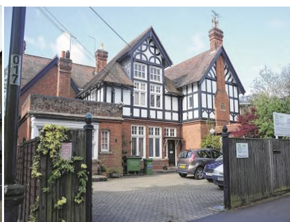
Photo 3 Essex Lodge Osborne Road
